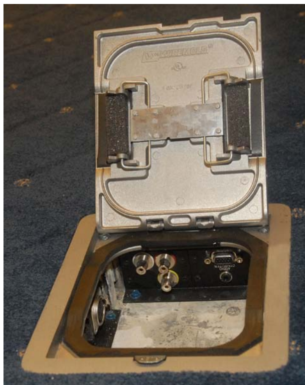
Figure 1. Computer and Audio/Video Connection Access in Floorbox
